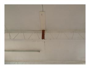
Leakage through brickwork due to ponding on roof area 3.
