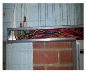
Current electrical cables installation throughout the building, utilising a mixture of MICC and PVC/PVC cables. Evidence of jointing of cables, dated cable colours and poor condition.
