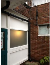
Office areas G224-232. Example of cracking to soffit with evidence of potential continuing movement.
