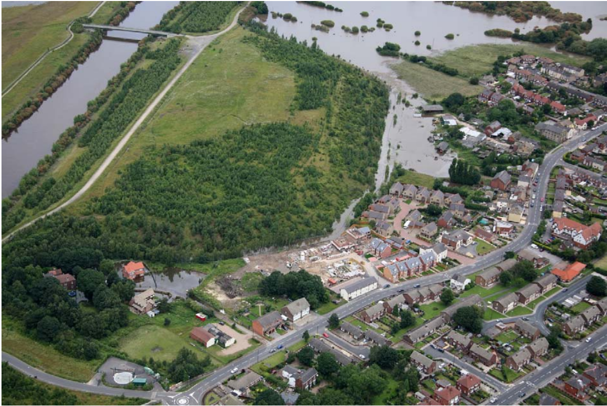
Figure 1 – Flooding at Mickletown in 2007
