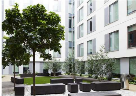
Light finish to external walls to maximise reflected light into the courtyard
