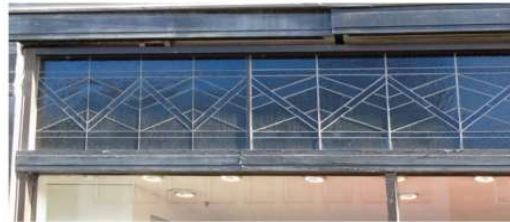
Image of Existing building detail at Ground floor level
