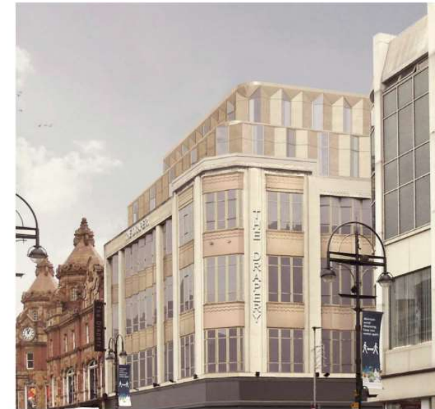
Proposed cladding amended at head of level 4 to improve transition between old and new
