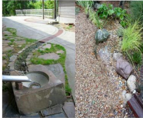
Disconnected downpipes
