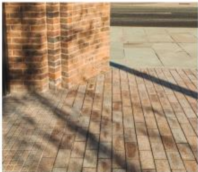
Small format paver in key locations - building thresholds
