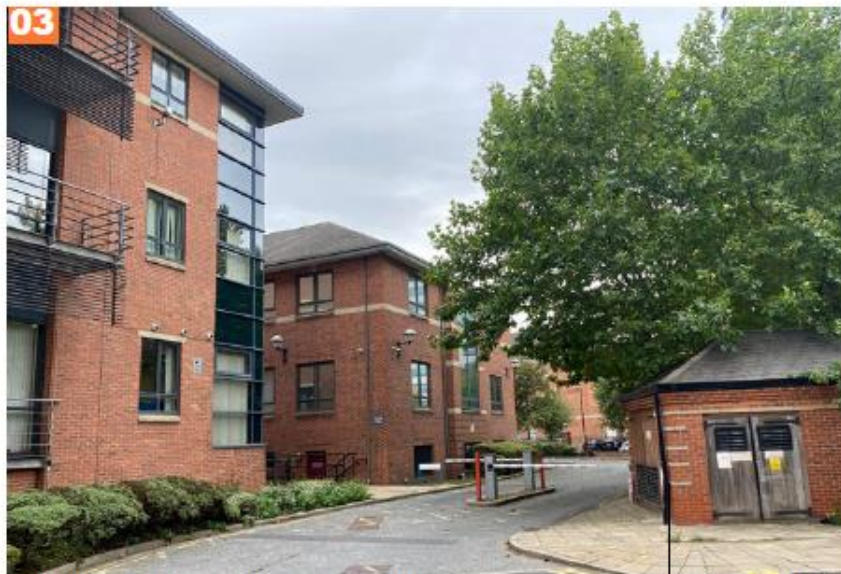
VEHICULAR ENTRANCE TO ZURICH HOUSE
