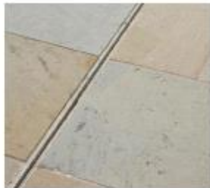
Yorkstone to pavements
