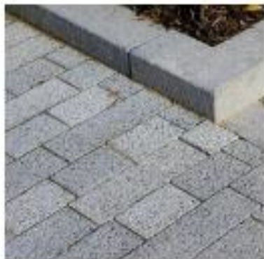
Quality Concrete Paver to pedestrian routes
