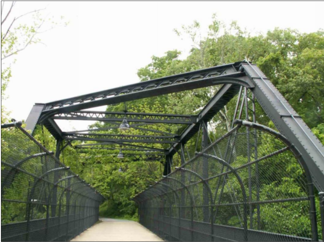
Photo 8 – 10 Years After Application of Termarust
