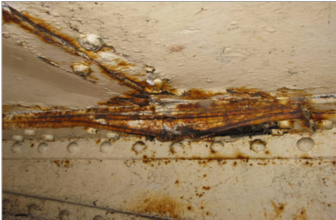
Photo 2 – Example of “Pack Rusting” on Leeds Bridge
