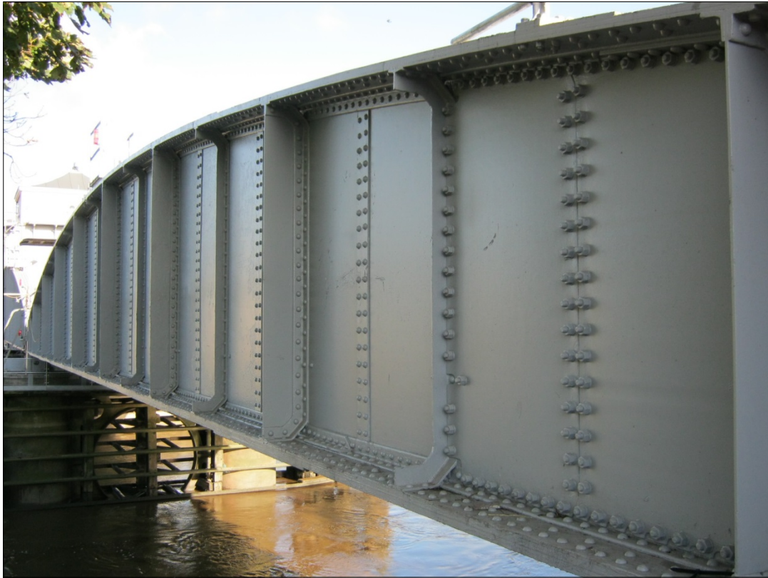
Photo 11 – After Application of Termarust
