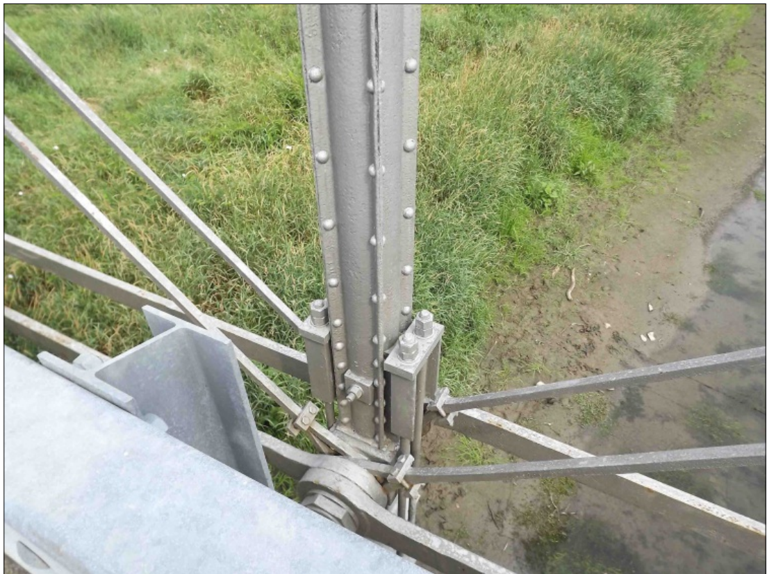
Photo 5 – 8 Years After Application of Termarust
