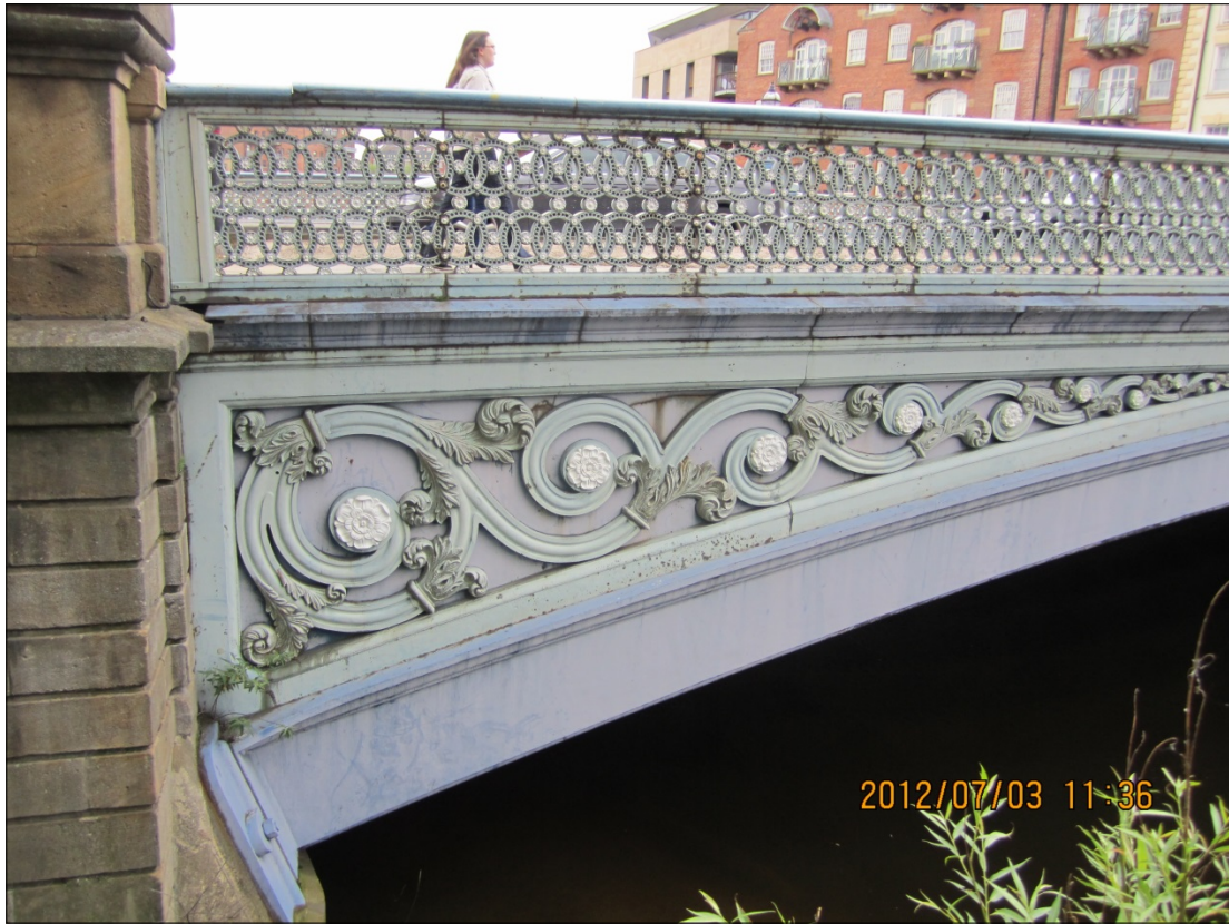
Photo 1 – Faded Condition of Paintwork on Leeds Bridge
