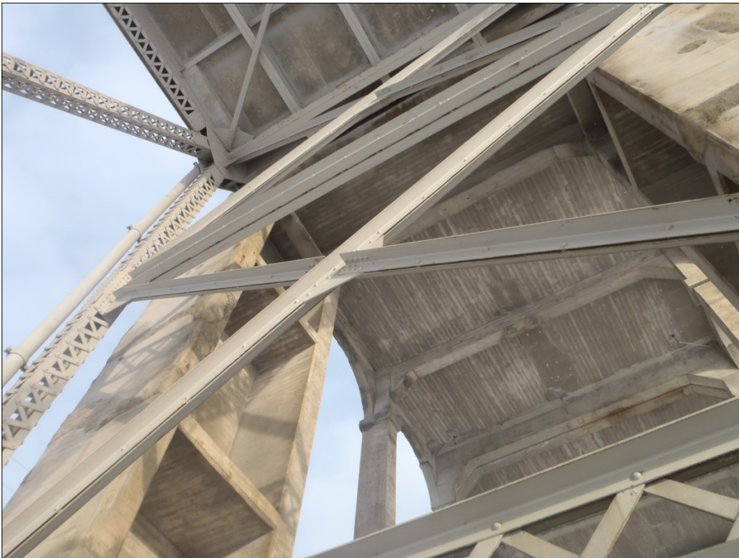
Photo 7 – 10 Years After Application of Termarust
