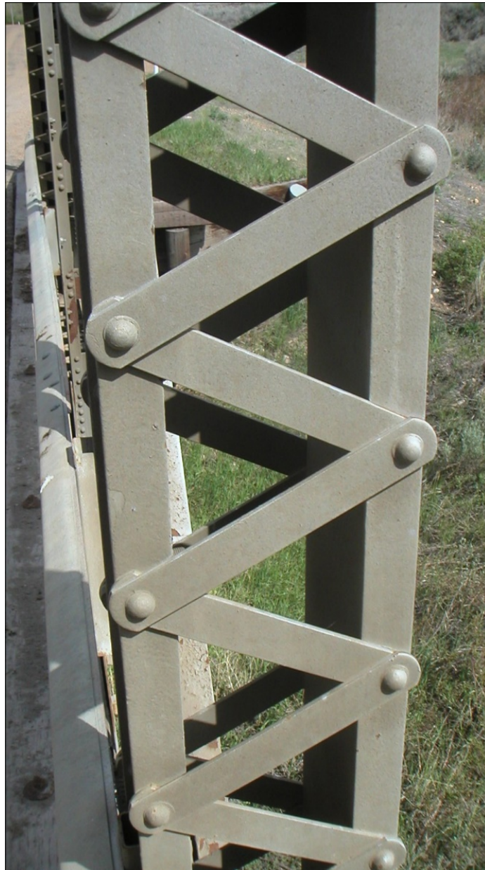
Photo 10 – 22 Years After Application of Termarust
