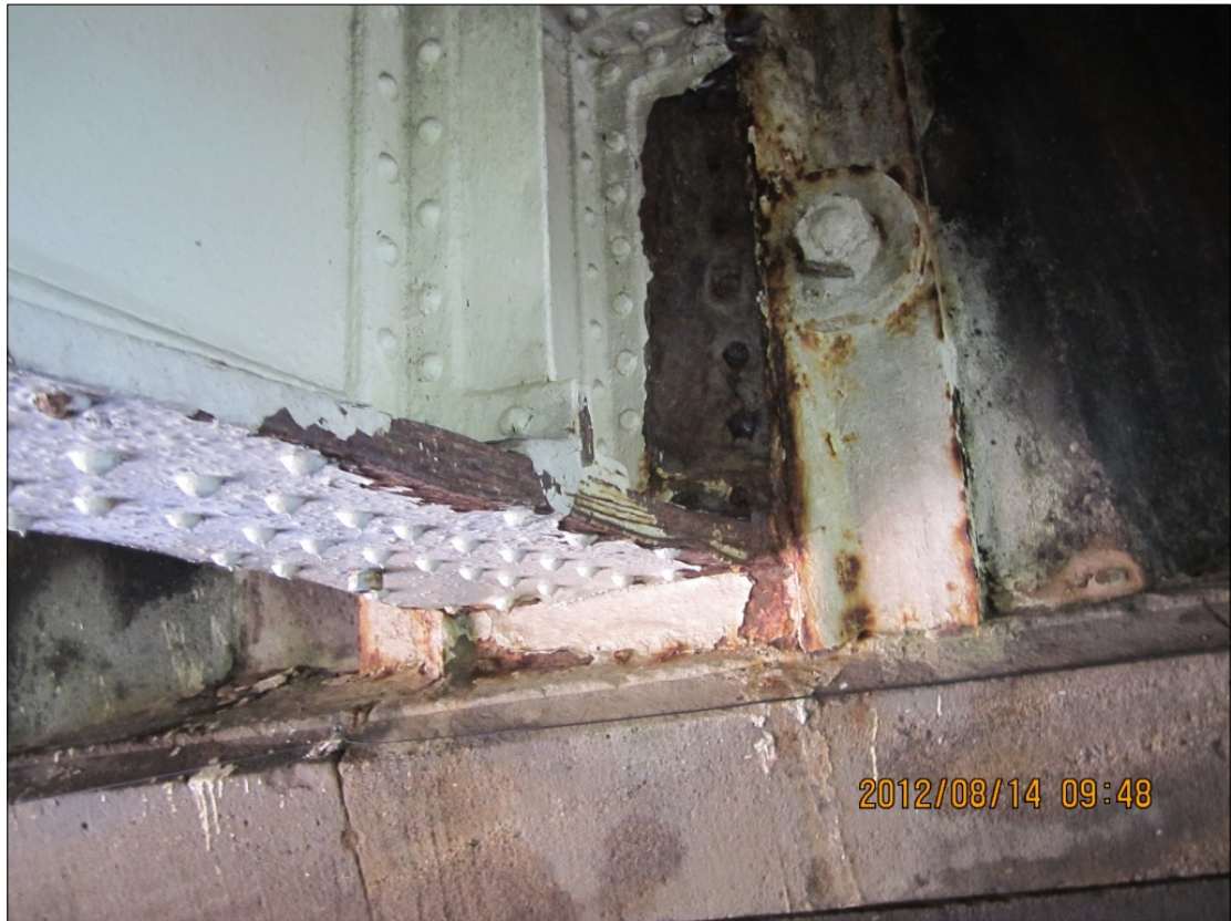
Photo 3 – Example of “Pack Rusting” to Main Arch Beam at Leeds Bridge
