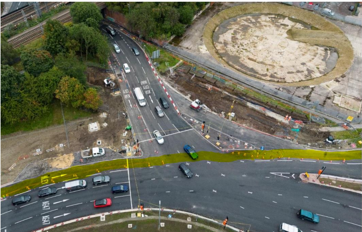
Figure 1 New (second) lane exiting the Gyratory towards Wellington Road (coned off)
