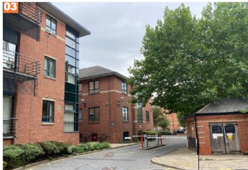
VEHICULAR ENTRANCE TO ZURICH HOUSE
