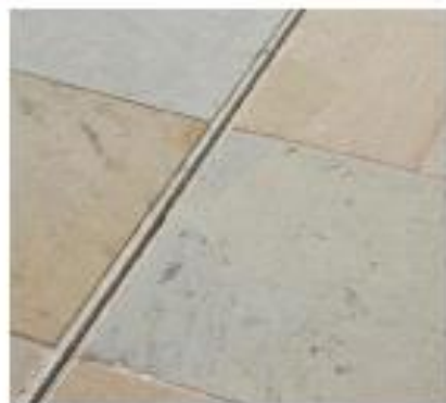
Yorkstone to pavements
