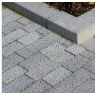
Quality Concrete Paver to pedestrian routes
