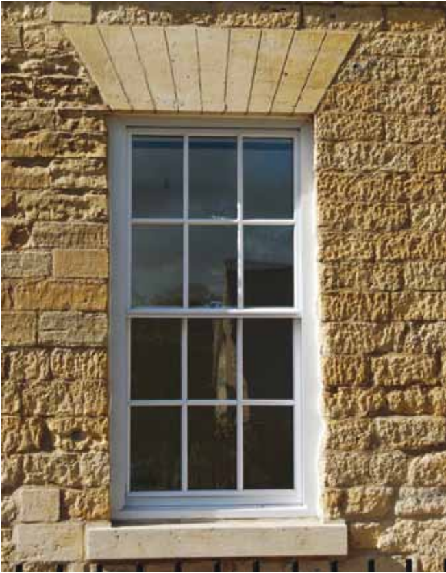
▲ Window details vary from house to house and it is important to make sure the windows in an extension reflect those of the main house ▶
