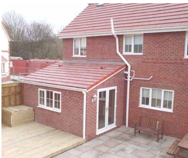
This extension has a simple shape and form and is of a modest size and scale. The use of matching materials helps to ensure it blends well with the house.
