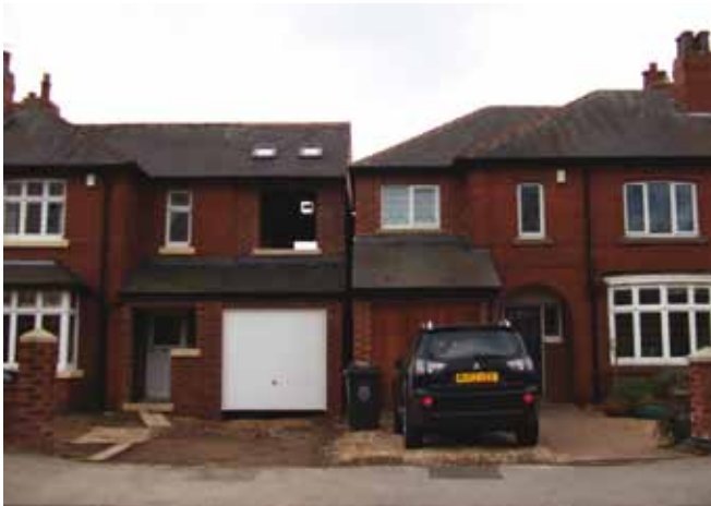
These two side extensions are built over the driveways of the houses and have wholly closed the gap between the two buildings.
