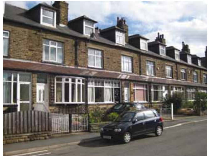
These dormers are small additions which are well positioned in the roofscape and do not cramp the chimneys. They sit above the existing first floor windows, use appropriate materials and are suitable to the age and style of the house.
