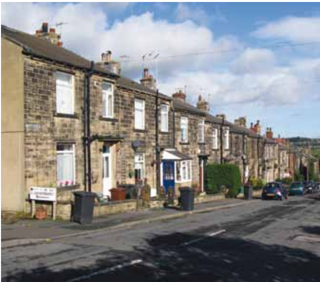
The clean, unbroken roofline of this terrace is an attractive part of the streetscene. The introduction of a front dormer would interrupt the simplicity of the buildings and would harm the character of the house and the wider area.
