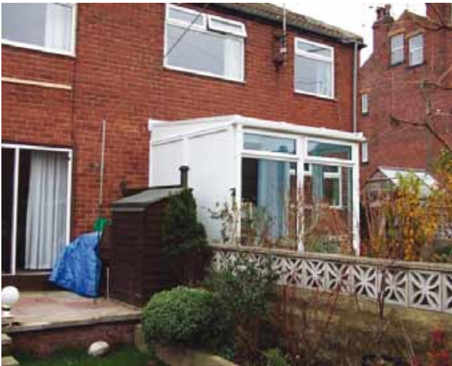
The use of obscure glazed or solid side panels prevents the neighbouring garden being directly overlooked.
