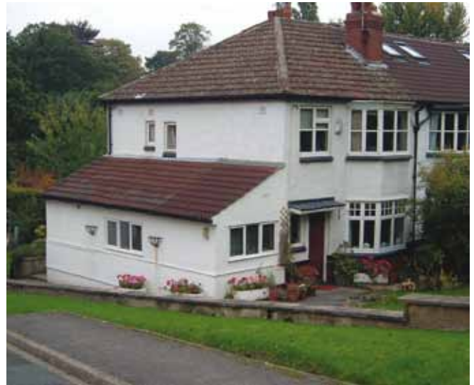
Even for a single storey extension it is important to get the details right. The wrong roof form can result in an extension which harms the appearance of a property.
